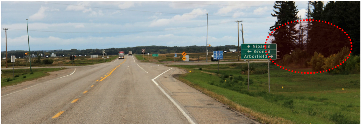
Highway 35 Northbound Approach (August 2018)
