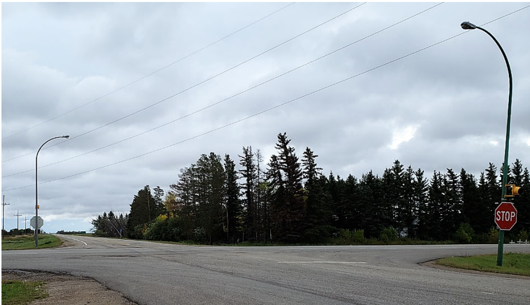
Figure 6-7: Highway 35 and Highway 335 Intersection Illumination
