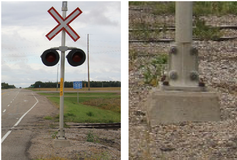
Railway Crossing Signals Within Clear Zone on Highway 35
